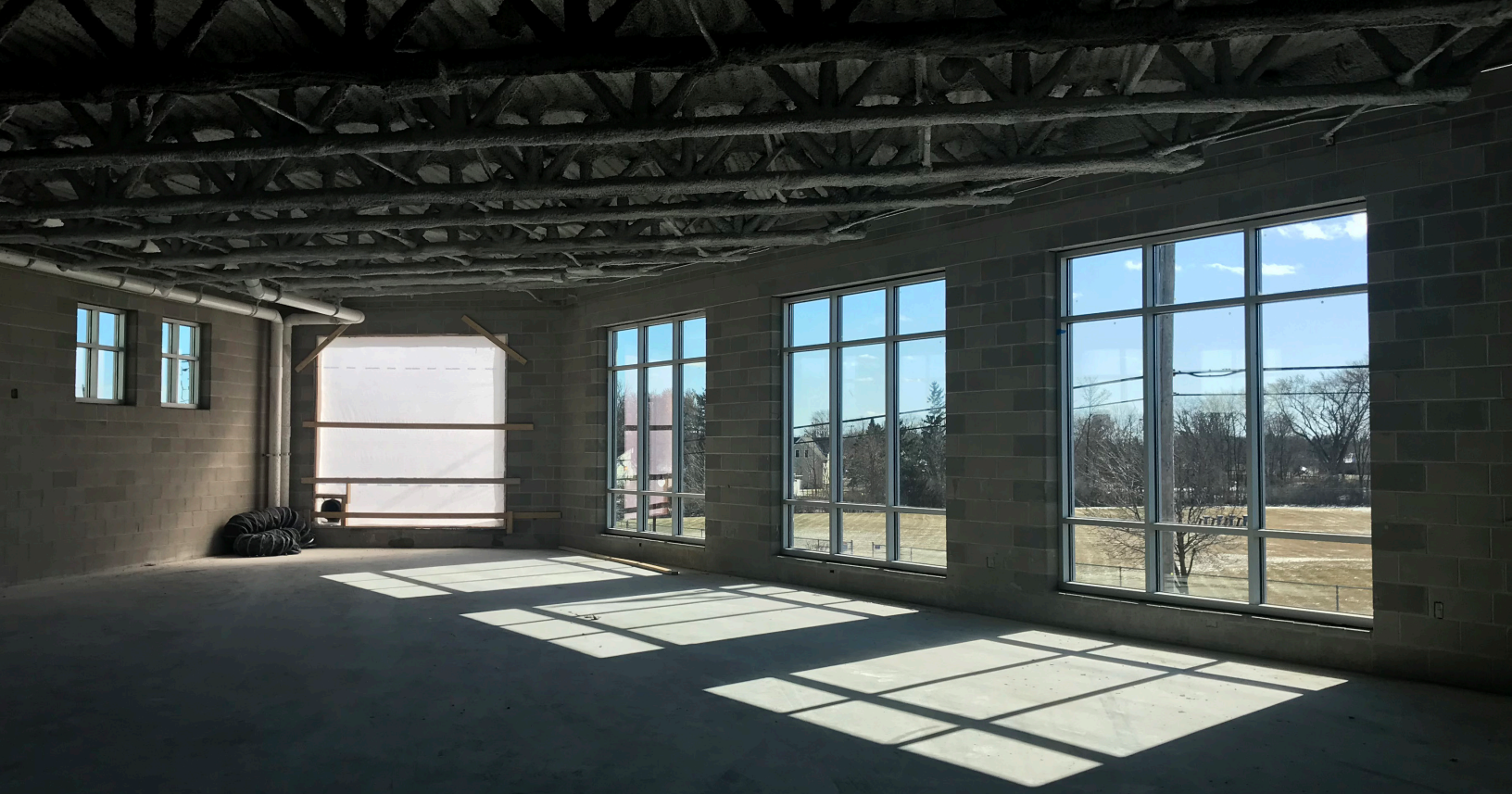
HORACE MANN HIGH SCHOOL | NEW WRESTLING & FITNESS ROOM
