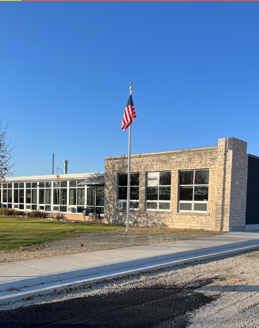
EARLY LEARNING CENTER | EXTERIOR FACADE
